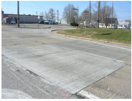
resealing performed on this CPR project. A total of 9053 SY of 9.5' thick PCCP was hand placed, finished with a straight edge, and properly tined. INDOT added some additional quantities during the project extending the original completion date by two weeks. The project began in mid-September and was completed at the end of November. Total project cost was \$1.12M and PCCP costs were \$787,500.
